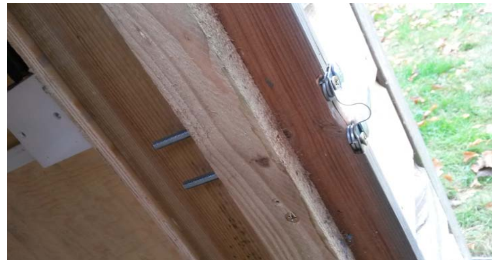
The bolts are now secured by long coach bolts
