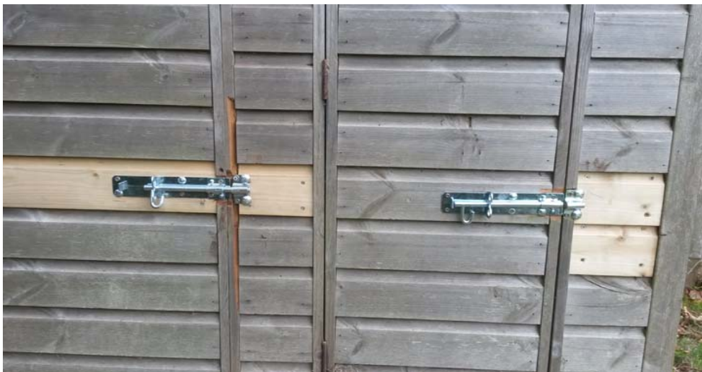
Repair of the Pavilion Services box following vandalism attack
