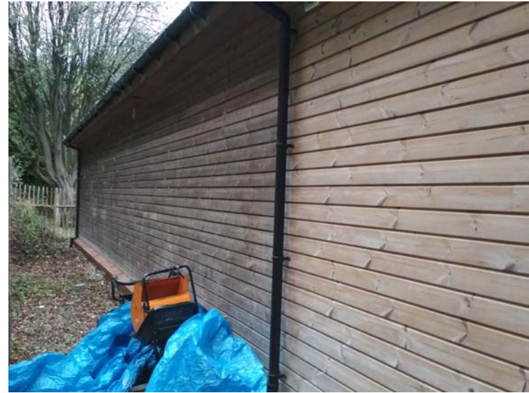
Cleaning of the wooden cladding at the back of the Pavilion with oxy-bleach ready for a coat of micro porous sealant. The front was completed last year.
